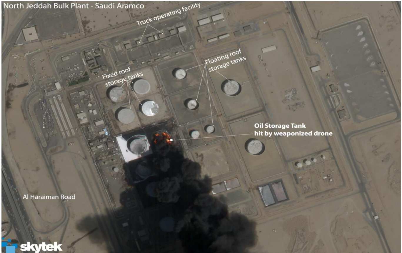
Figure 2 - Saudi Aramco's North Jeddah storage facility on March 26 th , 2022, showing a storage tank hit by a weaponized drone
