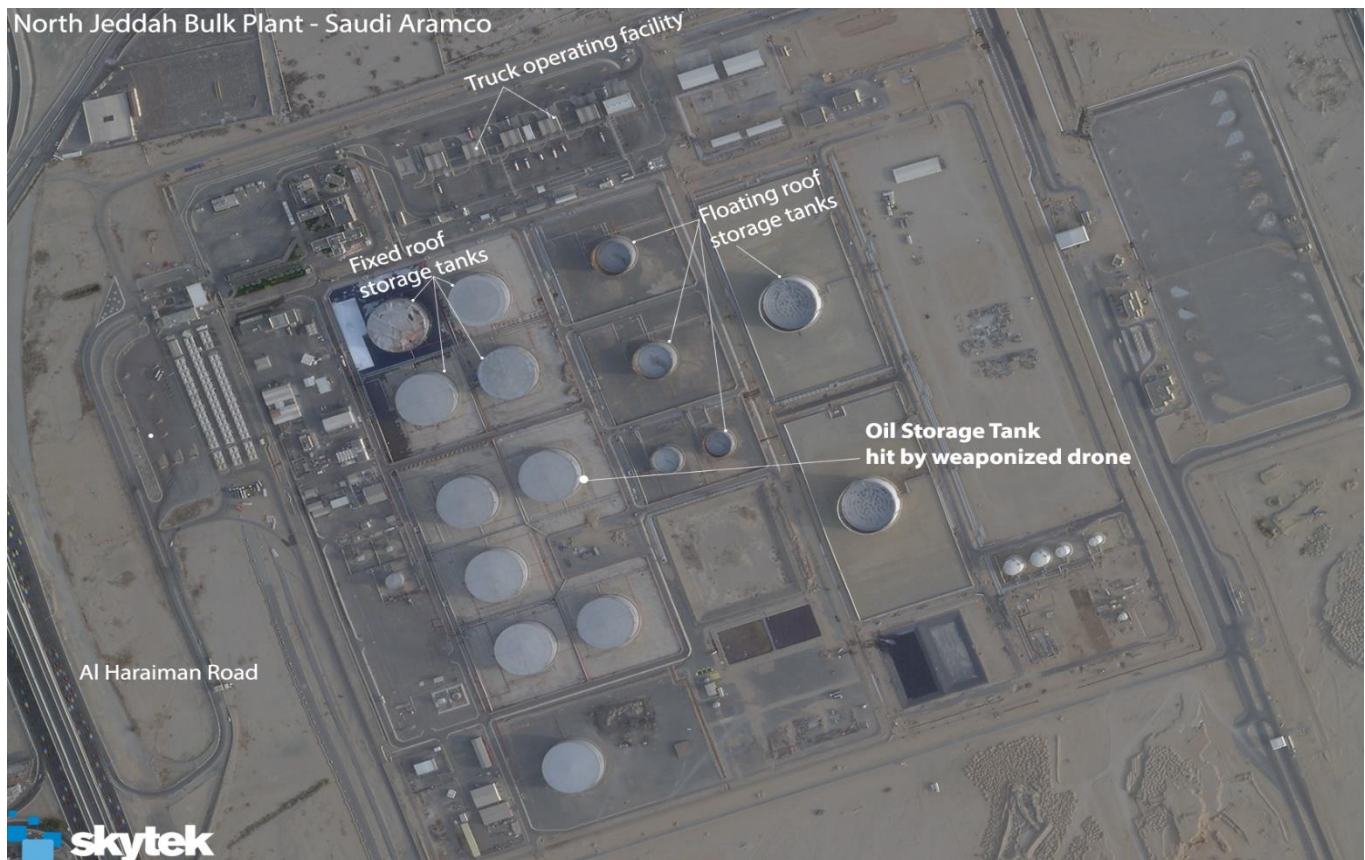
Figure 1 - Saudi Aramco's North Jeddah storage facility on March 22 nd 2022
